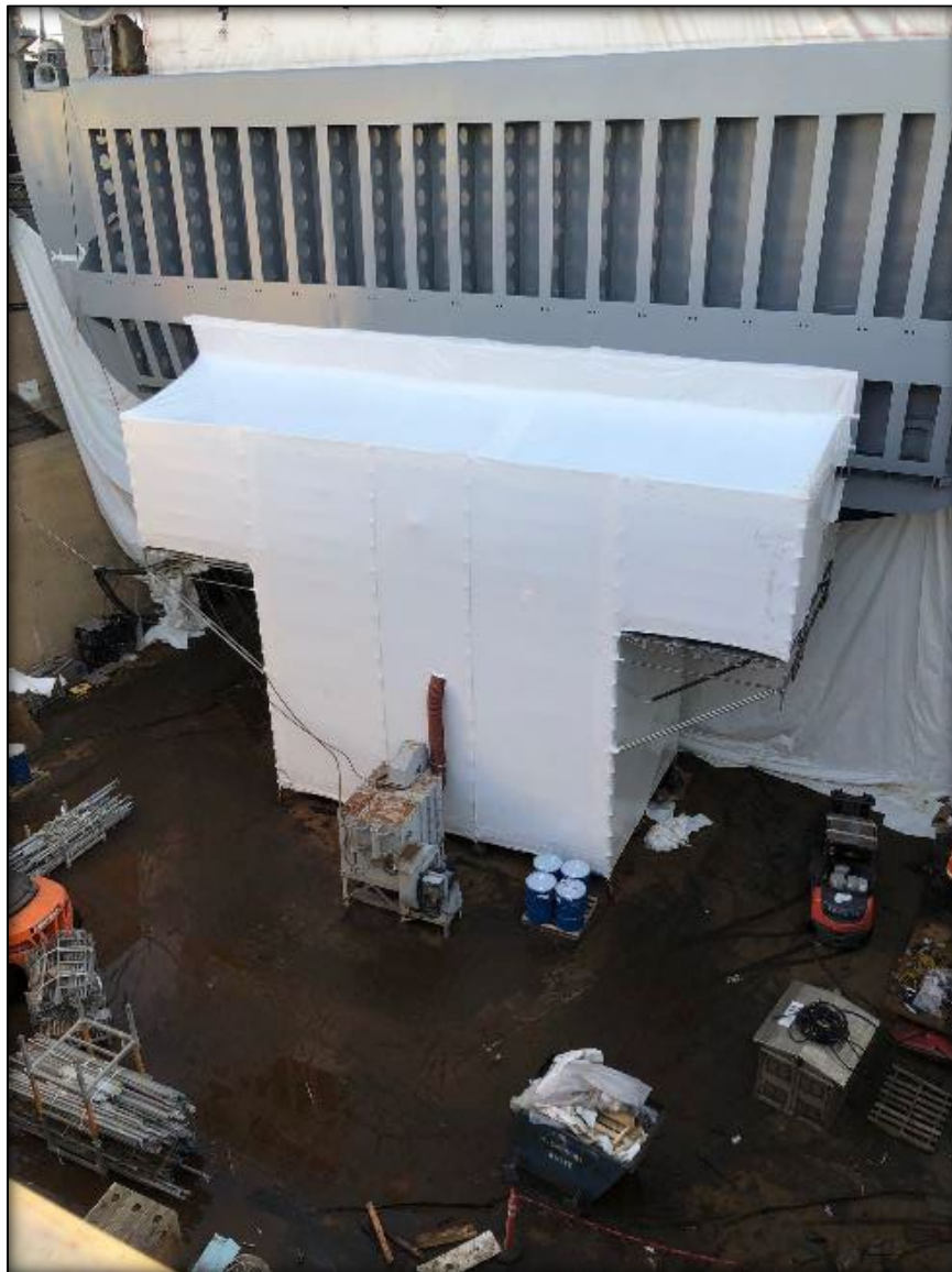
Figure 3-2. Installation of Ship Shrouding
