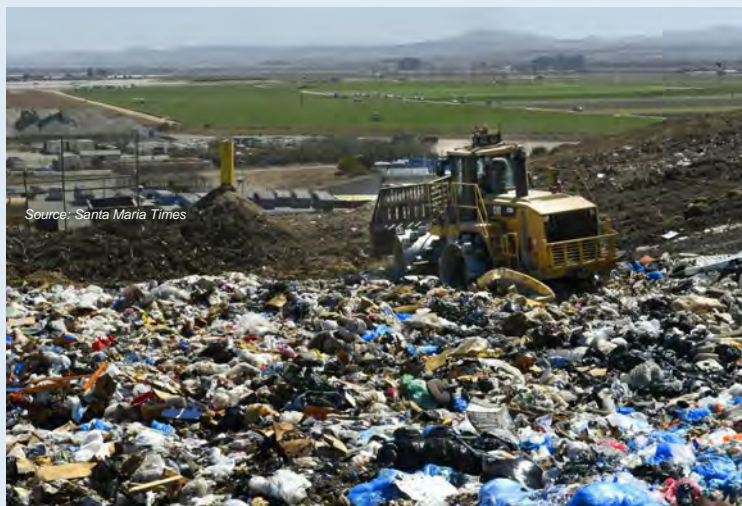
Collecting emissions from landfills is a complicated process, regulated at all local, State, and federal levels of government
