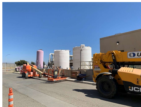
Tanks delivered on Aug. 18 for Chemically Enhanced Primary Treatment
