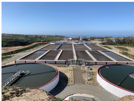
SAB WWTP, April 2025
