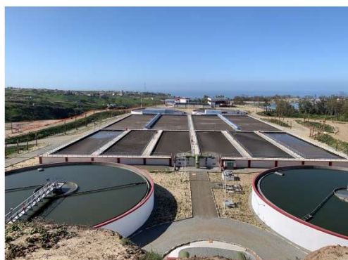
SAB WWTP, April 2025
